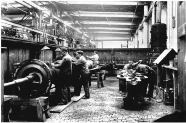
Fig. 2 Steam turbine assembly, Baden ca. 1902
